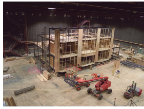
Picture 3 The real set construction
